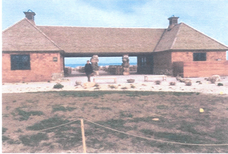
3. View Looking North Towards Old Barn, 2016
